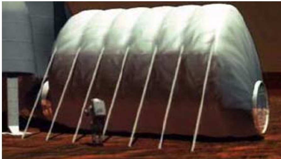
Figure 8: Pre-fabricated surface deployed hab unit
