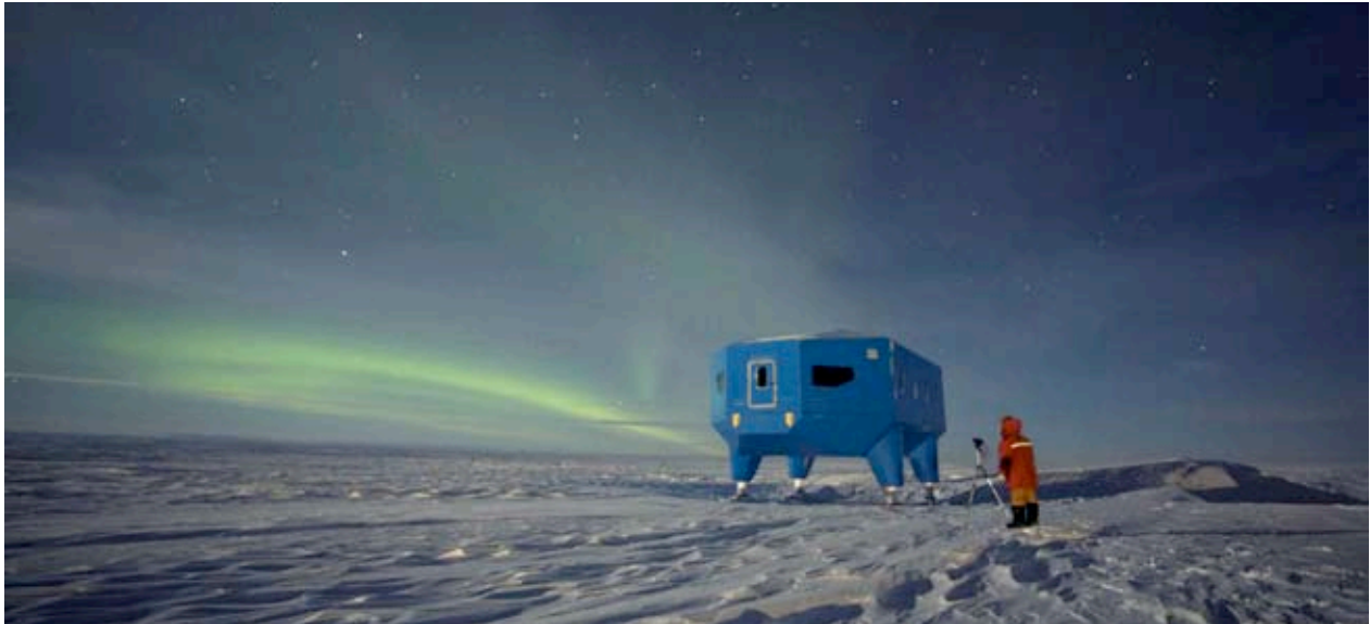
Figure 14. Halley VI module, seen against backdrop of the Aurora Australis – not so different to space?
