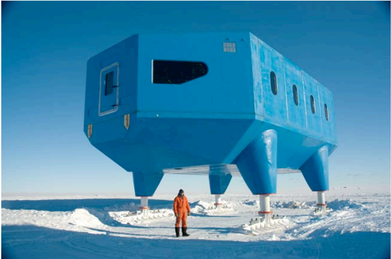
Figure 3. Completed module raised up on hydraulics ready to withstand its first Antarctic winter
