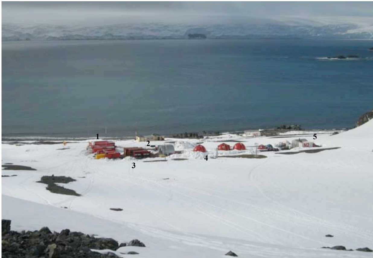
Figure 10. Existing Spanish Antarctic Base showing main habitat module (1), science labs (2), stores (3), sleeping pods (4), generators (5). Boat shed and fuel tanks are out of view
