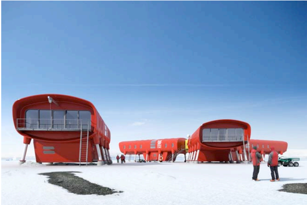
Figure 12. Balconies to ends of modules allow alternative means of escape and of entry at start of season. Glazing allows scientists to constantly engage with the stunning surrounding sea and landscape. In summer doors can be opened and scientists can use balconies for relaxation in the Antarctic sunshine.
