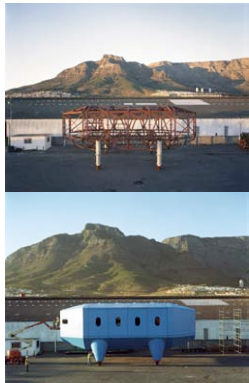
Figure 5. Test module erected in Cape Town as proof of concepts
