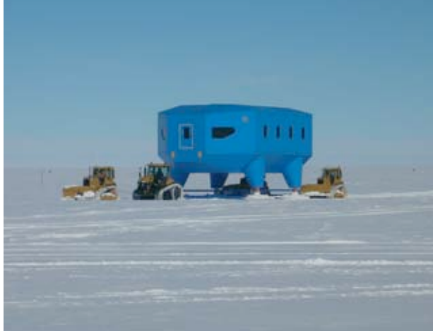
Figure 8. Relocating module with BAS plant
