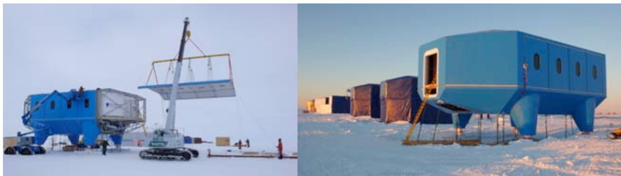
Figure 7: One module was clad with large FRP panels, while the others were temporarily protected in fabric
