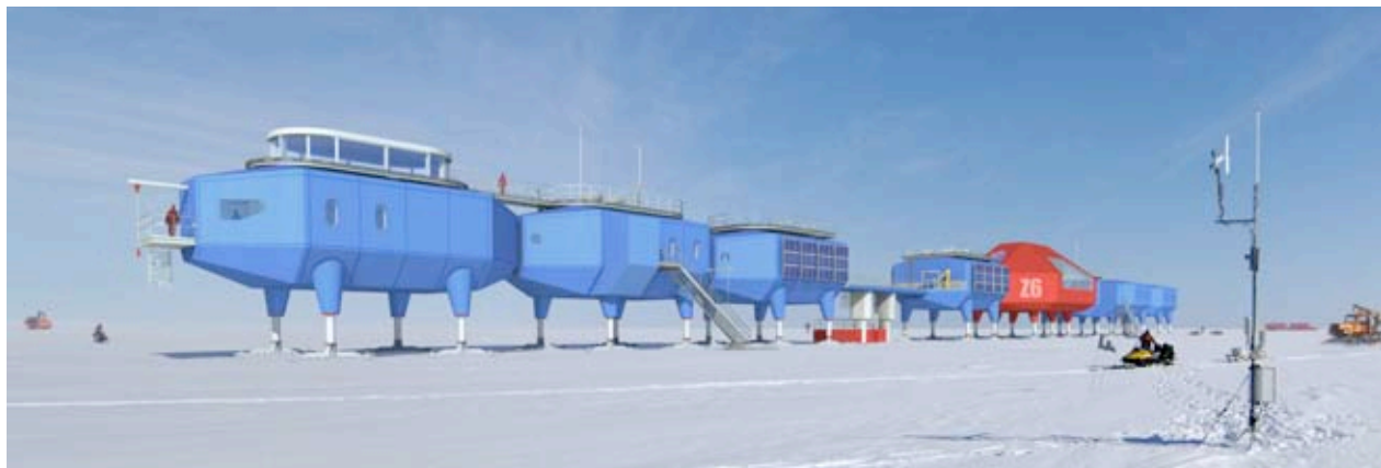
Fig 1: Visual of Halley VI with science modules in foreground and living accommodation in background
