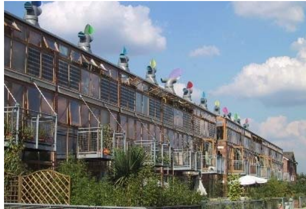
Figure 5. Image of BedZED 41 (UK). The project uses only energy from renewable sources generated on site
