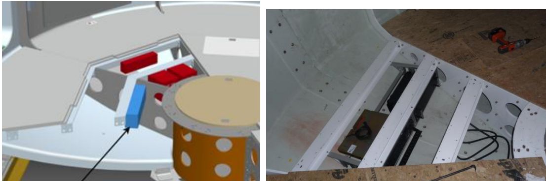
Figure 8 – At left, long red box was proposed terminal box location. At right, the absence of the terminal box at the planned installation timeframe
