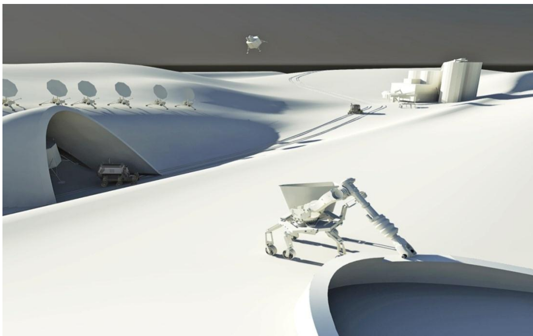
Figure 7. A Lunar CC System building an unpressurized storage hangar. A beneficiation plant that produces various feedstock from lunar regolith may be seen in the background. The lunar electric rover with a trailer cart would carry the feedstock in sorties from the plant to replenish the CC machine.(credit C.Wingfield, B.Farahi)
