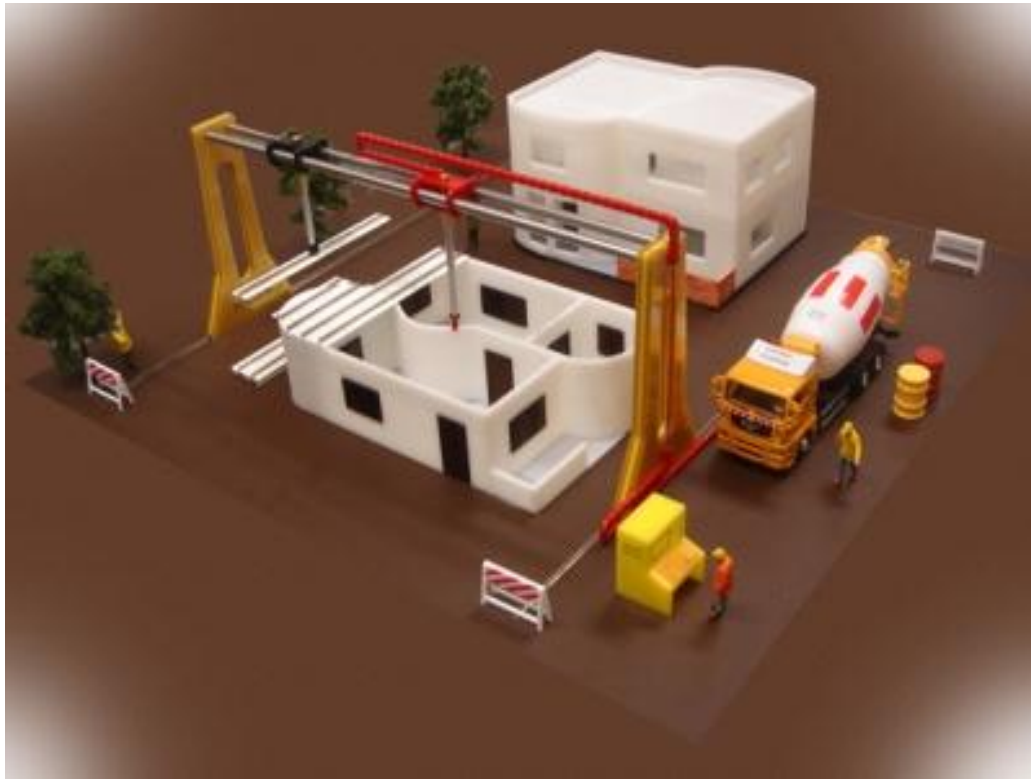
Figure 5g. Classic Contour Crafting gantry building a terrestrial multistorey structure Figure 5h. Hybrid options using all or some of the above in concert.(not depicted)
