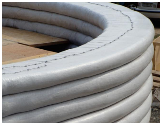
Figure 7B: Cal Earth (SuperAdobe) layer by layer deposition construction method.
