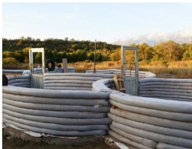
Figure 7B: Cal Earth (SuperAdobe) layer by layer deposition construction method.
