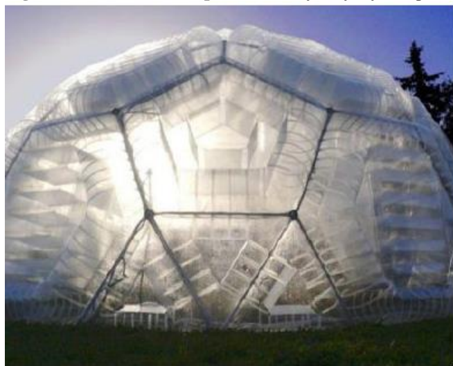
Figure 7C: Pneumocell: cellular membrane construction.
