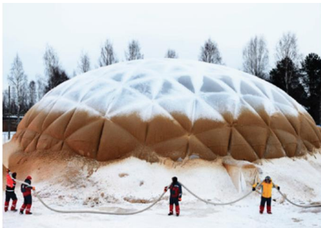
Figure 7A: Pykrete Construction: Inflatable Scaffold, Spray On. Thermal Control: Snow/air as insulation
