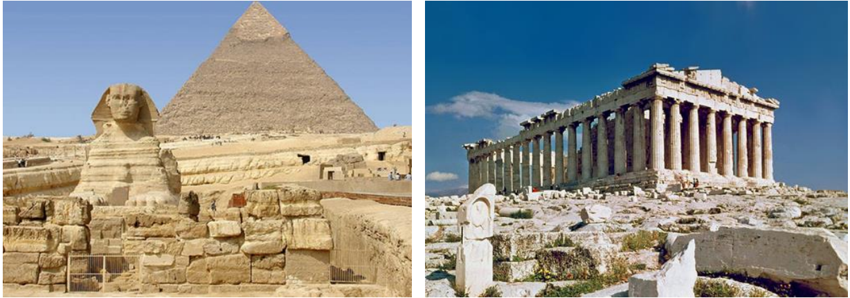
Figure 7a,b The Egyptian pyramids and Sphinx, shown in 7a (Bart), were built 4500 years ago, and the Greek Parthenon, shown in 7b (“The Parthenon”), from 2500 ago are rock structures that were built with hand tools and still possess structural integrity. The pyramids also have great insulation properties attributable to thermal inertia, holding steady internal temperatures during the extreme diurnal thermal cycles of the desert. This property could be an asset for extraterrestrial rock structures.
