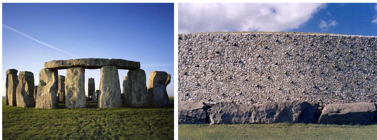
Figure 6a,b – Stonehenge, in 6a, is an example of a rock structure that was quarried and erected 2500 years ago (“History”). Dry packing technology at the 5200 year old Newgrange Tomb Wall, shown in 6b, show the capacity of handbuilt rock structures to weather the elements (Stout).
