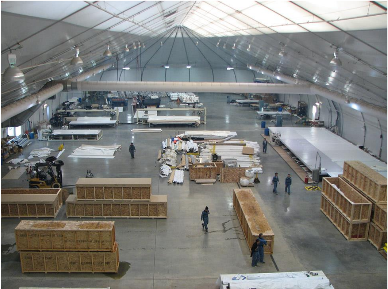
Figure 3. SPRUNG structures offer the possibility of quick deployment and very spacious, unfettered volumes that could prove useful for thermal and micrometeoritic protection on the lunar surface. By erecting pressurized inflatables within such structures, it is possible to combat and ameliorate the harsh lunar environment for crew in activities that extend the IOC activities of early crew.
