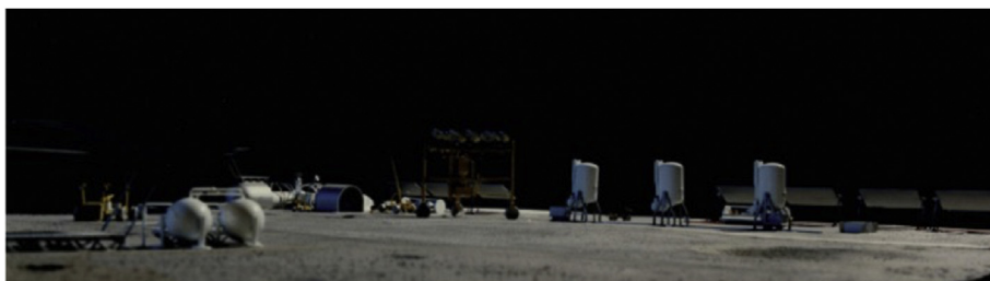
Fig. 7. Hydrogen reduction of ilmenite is a batch process , run with photovoltaic power during the two-week lunar day. The sealed reactors (right) cool down during the long night, are opened, emptied by the high-reach Truck, and readied with a new batch of feedstock. Oxygen product is piped to a liquefaction and storage depot adjacent to the landing pad (left).
