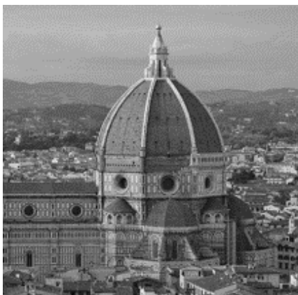
FIGURE 8. Brunelleschi’s Duomo of the cathedral in Florence, with the horizontal band of radial rondel windows and the cupola.
