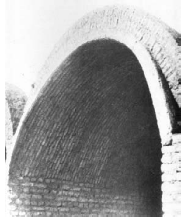
fig. 19 vault built using leaning arches
