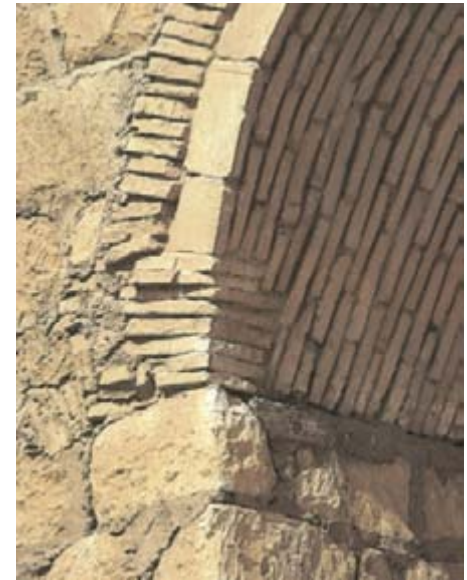
fig. 38 free end of a pitched-brick vault
