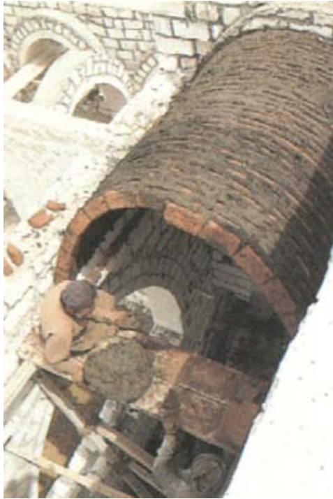
fig. 18 construction of a vault without centering
