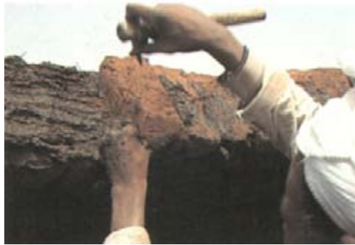
fig. 27 Constructing a brick dome using concentric brick courses in contemporary Egypt.
