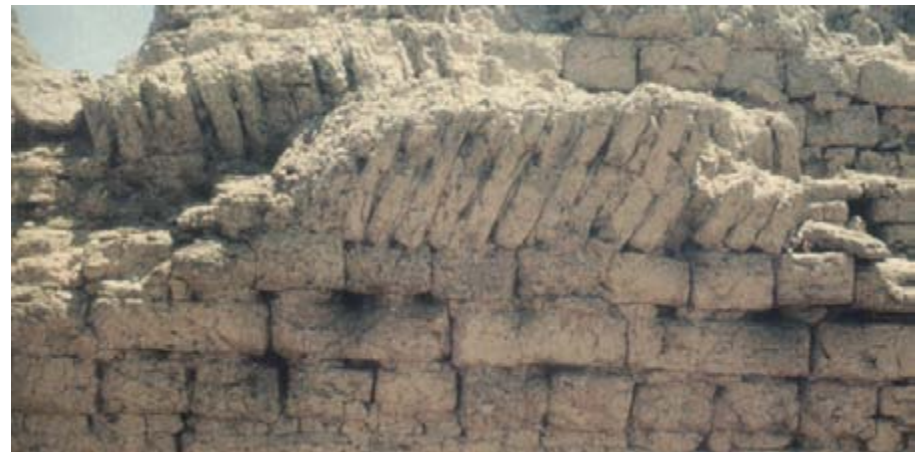
fig. 39 Detail of the vaults at the Ramesseum, notice the opposite pitch of bricks on alternating courses
