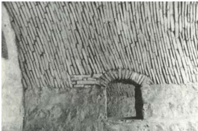
fig. 36 pitched-brick vault with opening
