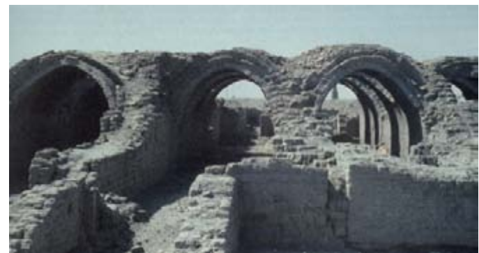
fig. 16 Vaults at Ramesseum, 13th century b.c. storehouses in Egypt. Each vault consists of four courses of mud brick. Successive courses lean in opposite directions. about 4 m span.
