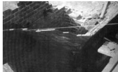
figs. 40, 41, 42 Catalan vaulting: thin tiles are arranged one course at a time to complete a large number of compression forms. Fast-setting mortar is required to hold the tiles in place until each course is completed.
