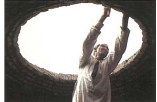
fig. 27 Constructing a brick dome using concentric brick courses in contemporary Egypt.
