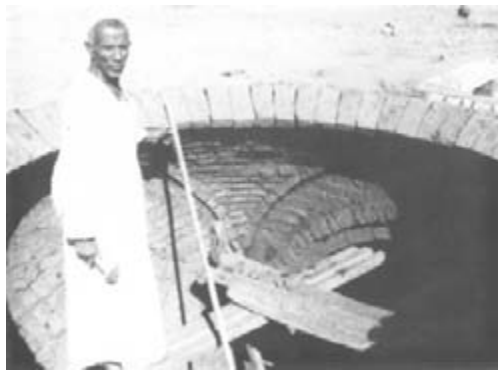
figs. 24, 25, 26 Steps in the construction of a masonry dome notice the measuring stick that is used to guide the geometry of the dome
